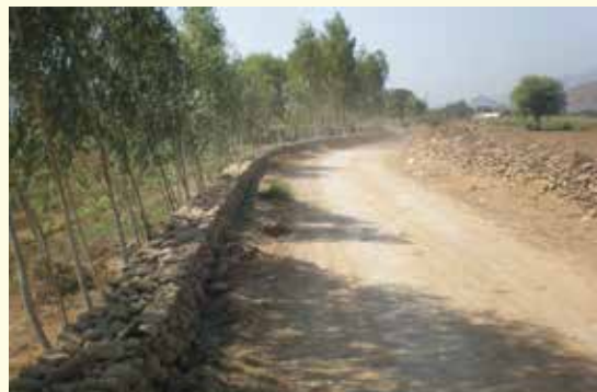
Condition of the road before and after widening and repair
