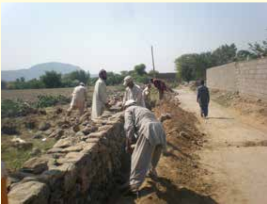
Condition of the road during and after widening and repair
