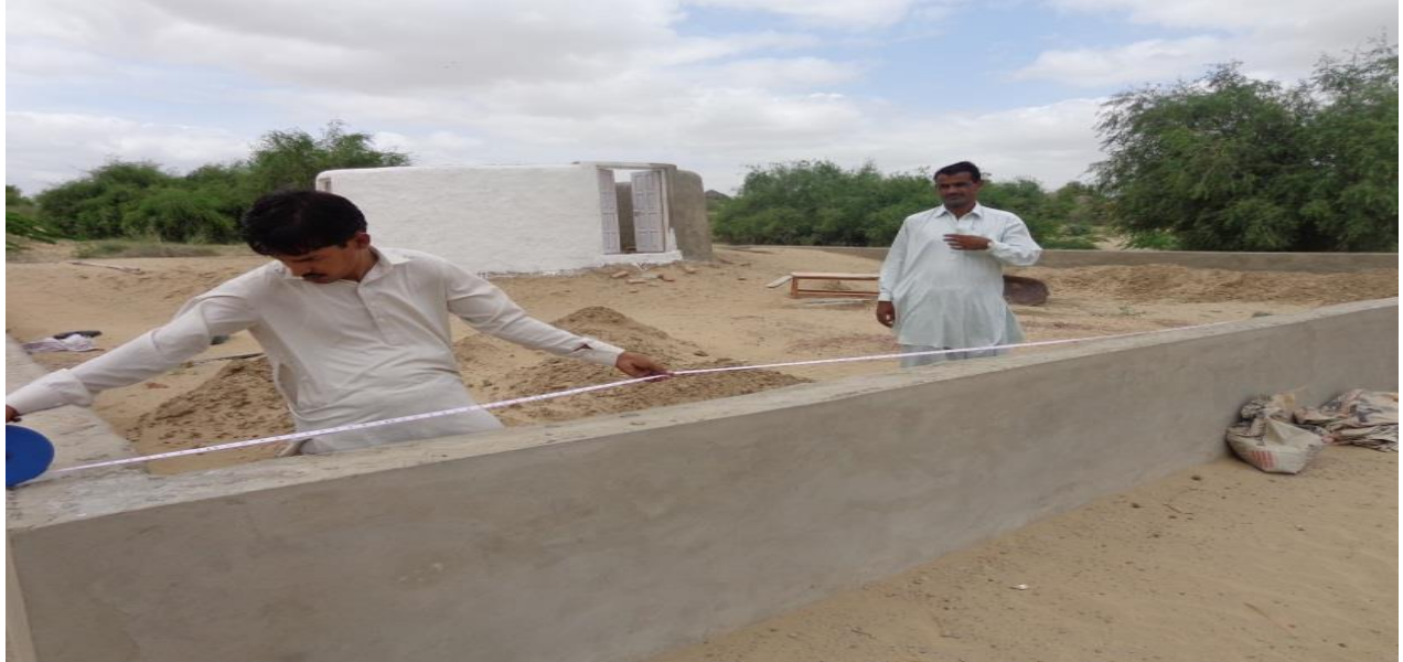
Construction of rescue point in progress
