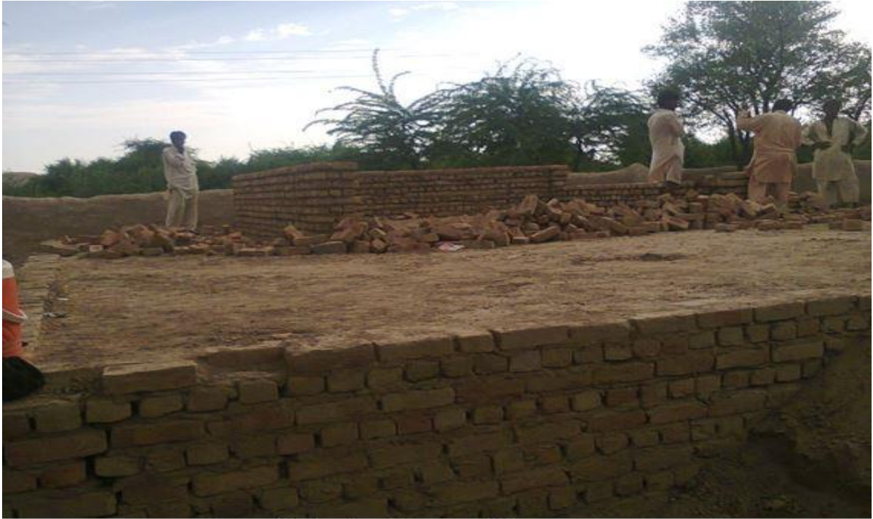
Construction of a rescue point in progress
