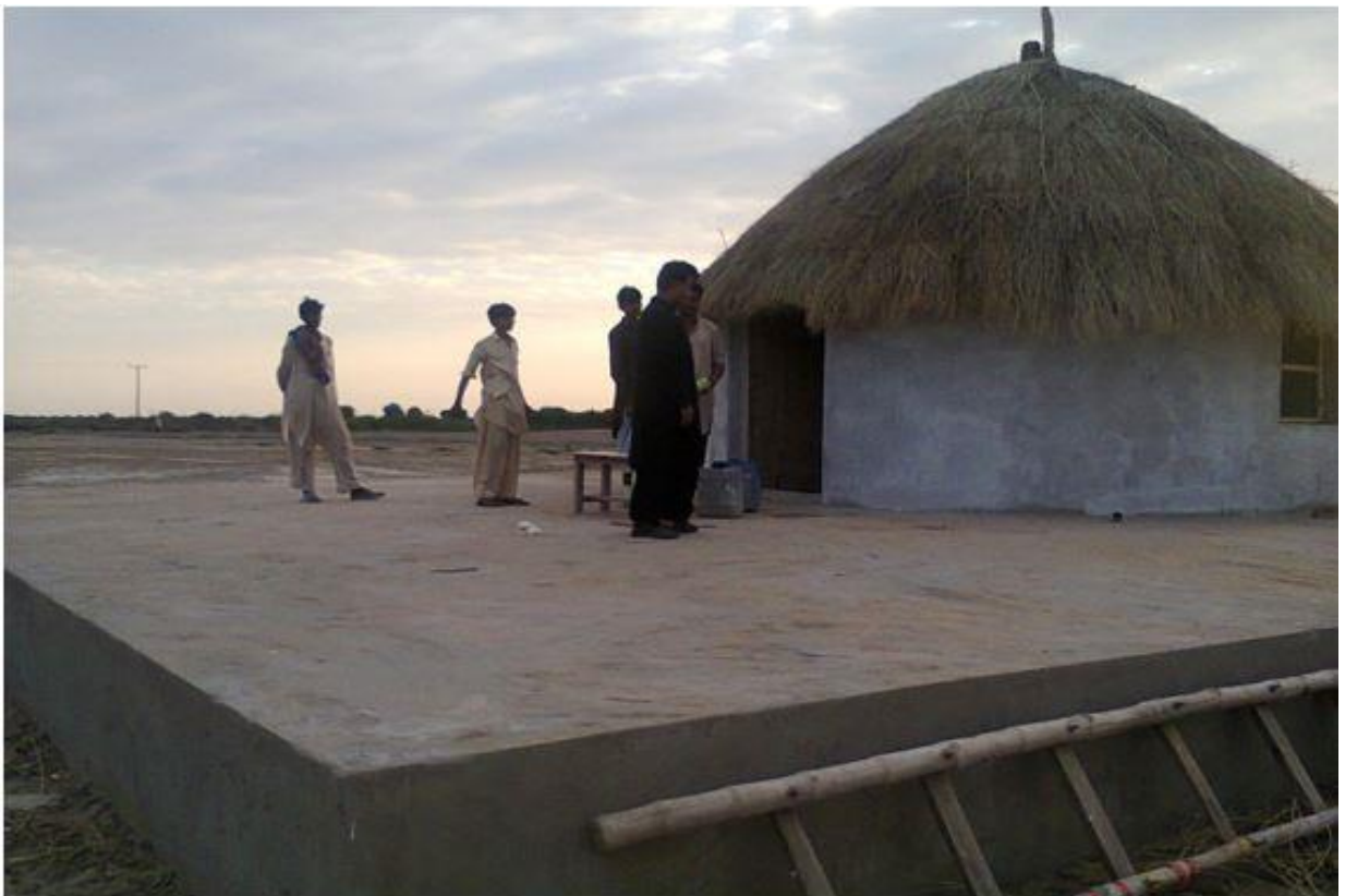
Rescue place completed at VDMC Kaith, Umerkot
