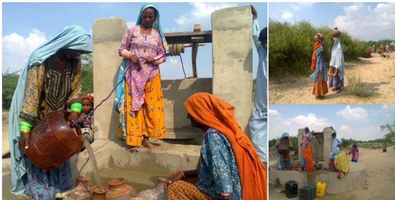
Women getting facilitated with a dug-well constructed in settlement Baheed Khan Khaskheli of Revenue Village Nabisar Thar of district Umerkot
