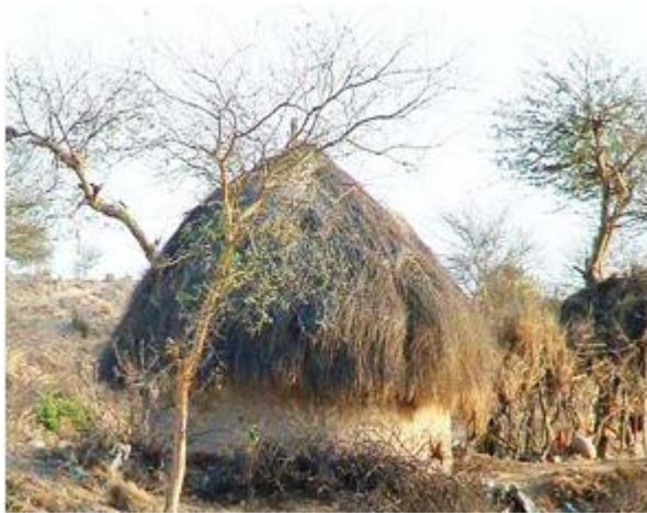
A Locally constructed house named as "Chowro"
