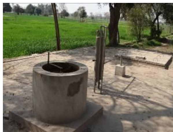
Biogas Plant constructed in Mirza Manzoor's Farms
