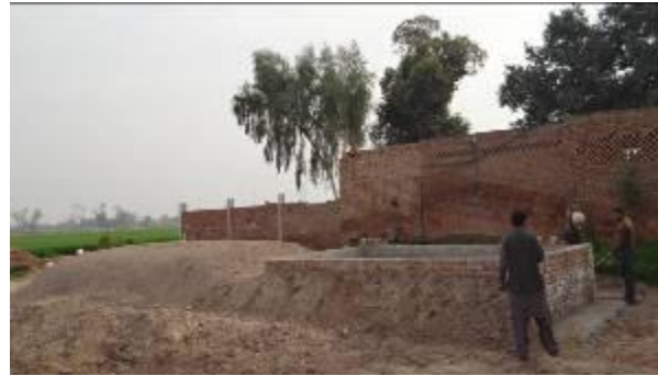
A new plant ( 50\text{M}^3 ) under construction for running Tubewell on Biogas
