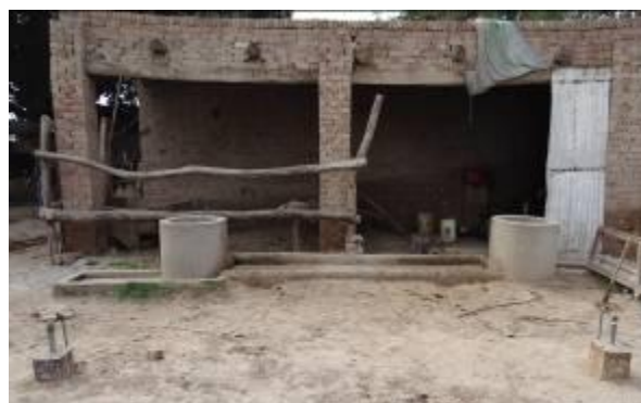
2 Biogas Plants (15M 3 each) constructed in Haji Irshad's Farm House
