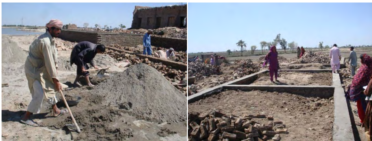
Construction of Transitional Shelter is going on
