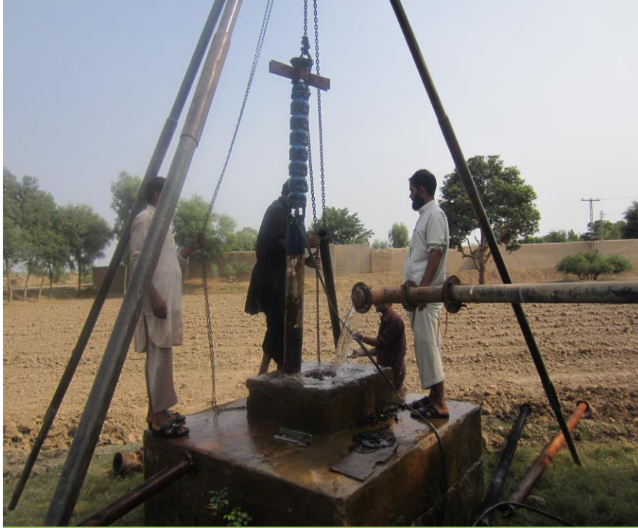
Scheme under repair
