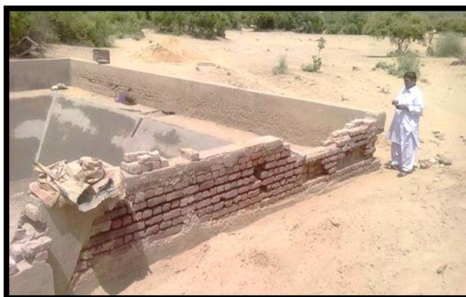
The damaged rain water harvesting pond being repaired
