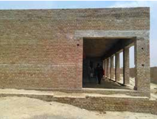
CONSTRUCTION OF NEW BUILDING IN BAHAWALPUR
