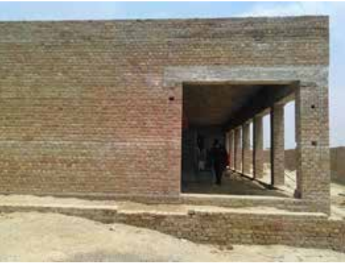
CONSTRUCTION OF NEW BUILDING IN BAHAWALPUR
