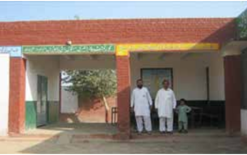
SCHOOL IMPROVEMENTS IN GOVERNMENT CENTRE PRIMARY SCHOOL, BASTI PAHORAN - BAHAWLAPUR
