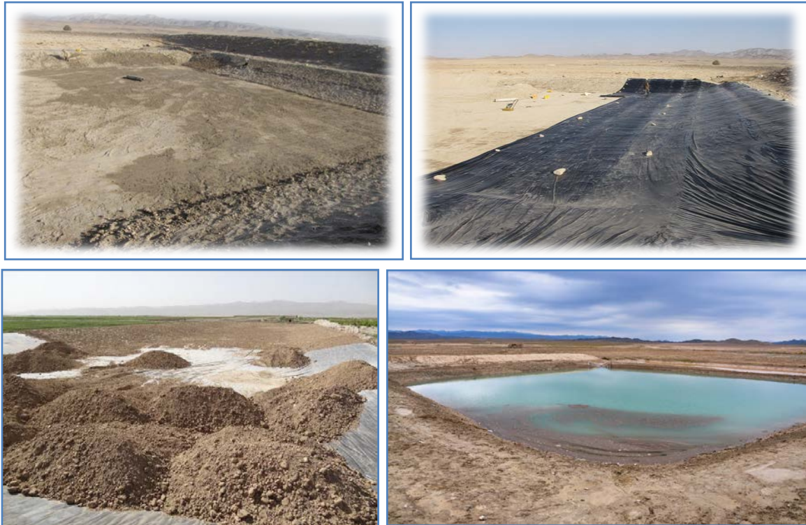
Figure 82: Rehabilitation of water storage tanks at the Iskan Khan Pilot
