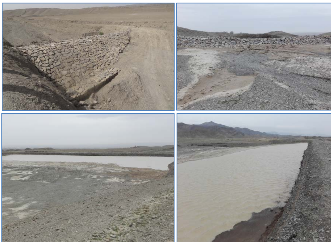
Figure 86: Check dams and desiltation of water storage tanks
