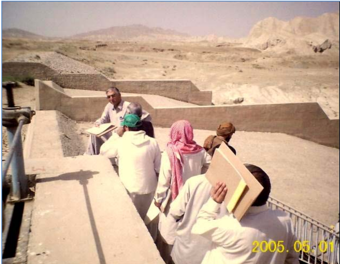
Figure 27: Un-gated weir controlled off-stream water diversion to water tanks
