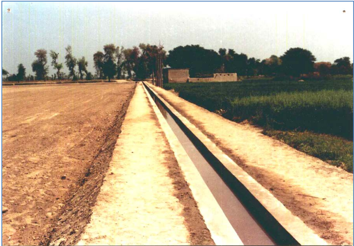
Figure 40: Improved lined watercourse
