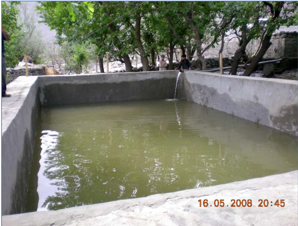
Figure 10: Storage of water in lined tank
