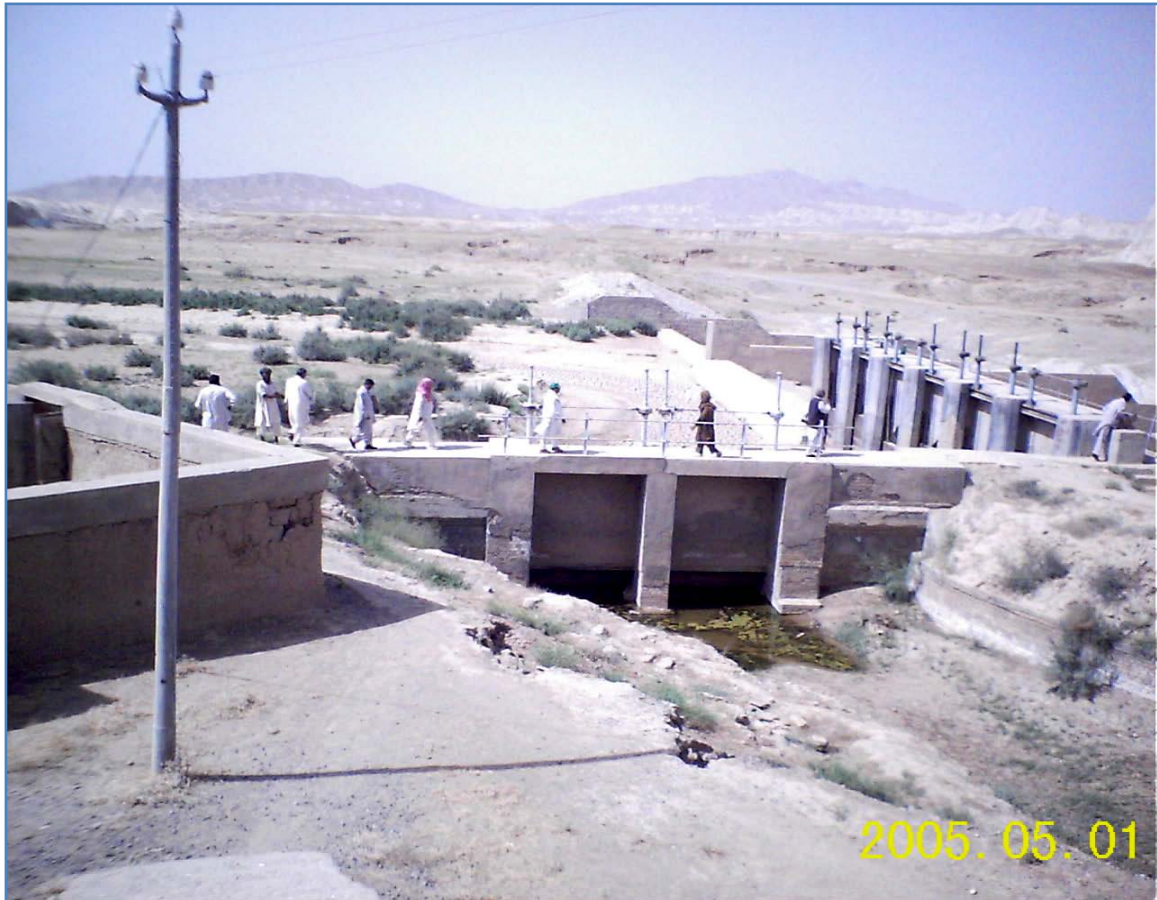
Figure 23: Weir canal at Shabo Headworks, Pishin district, Balochistan, Pakistan
