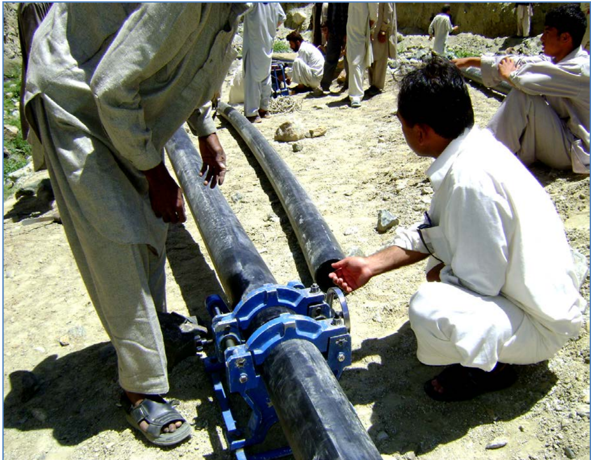
Figure 18: Heat welding of pipe by the Dadex Eternit Pvt. Ltd. Pakistan
