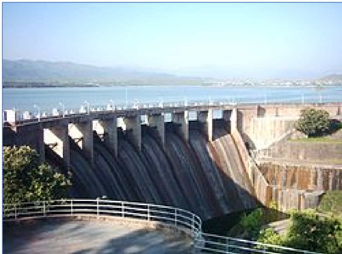
Figure 31: Spillway of the Tanda dam, Kohat District of Khyber Pakhtunkhwa
