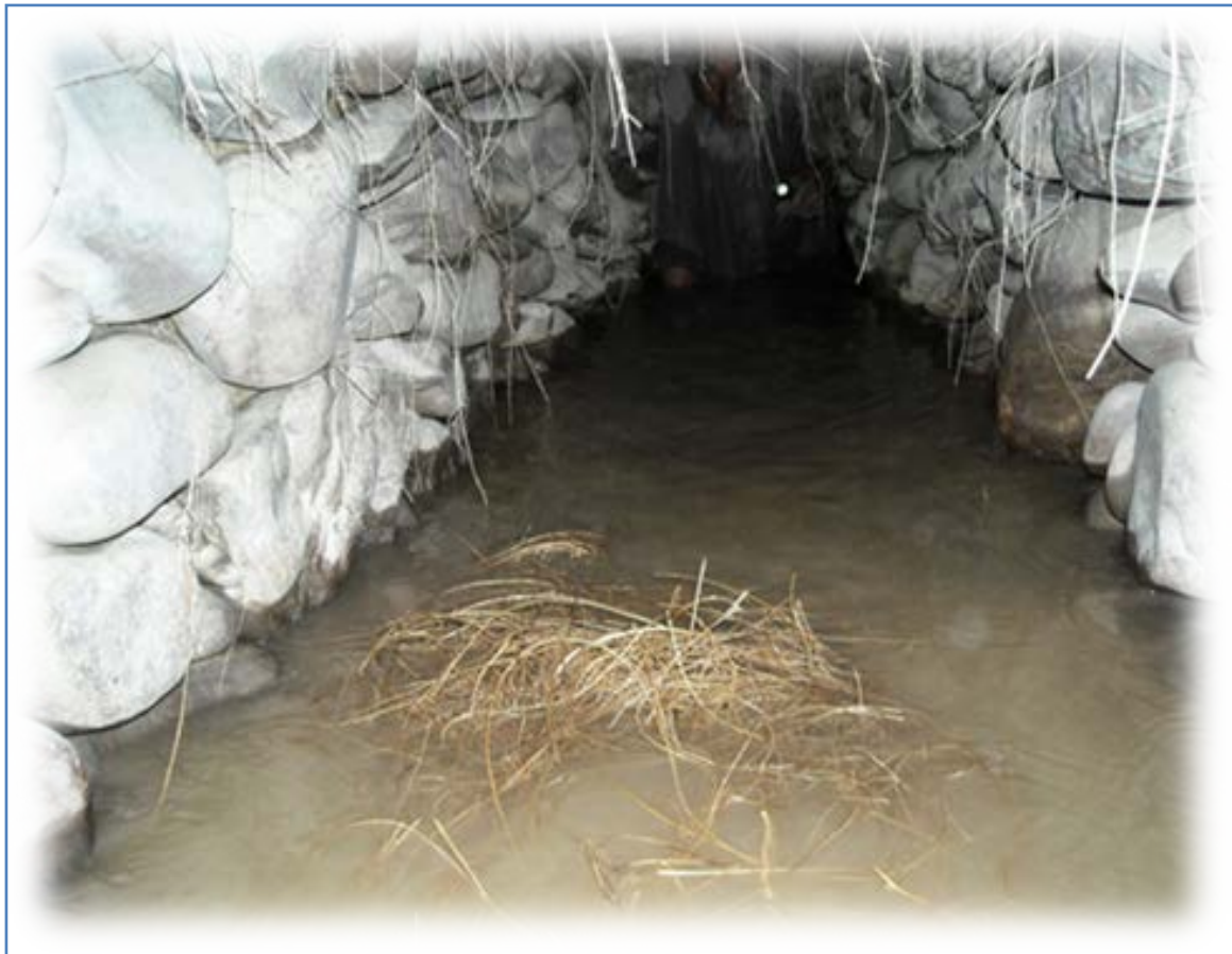
Figure 81: Cleaning of main channel upstream of daylight point
