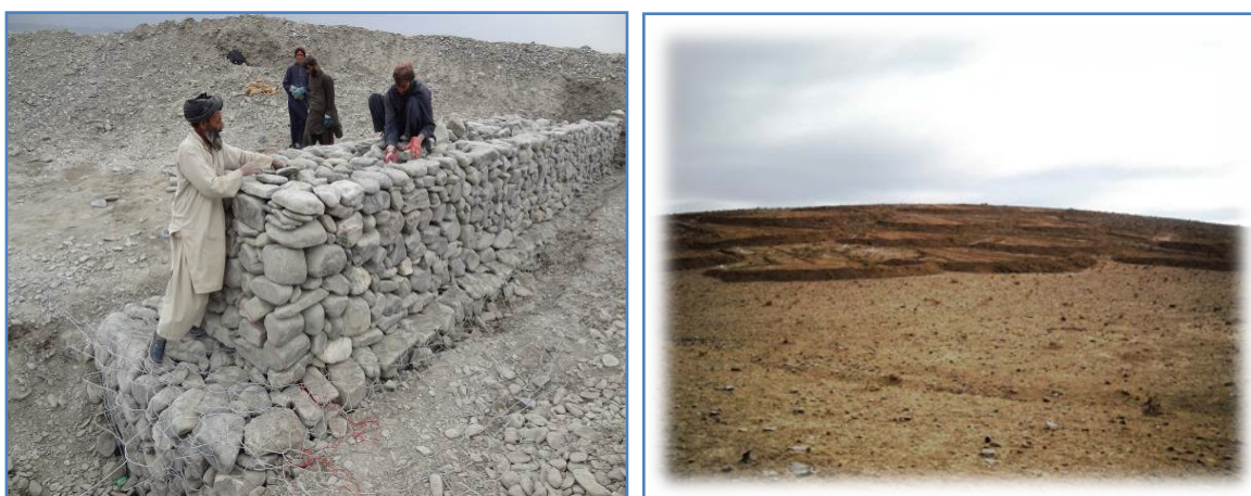
Figure 83: Micro-catchments and retaining walls in the Iskan Khan Pilot
