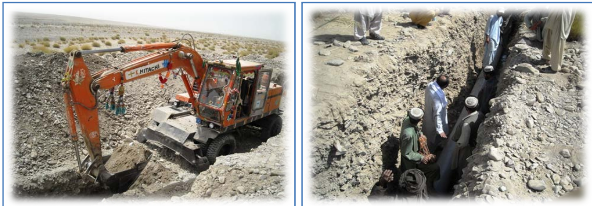
Figure 80: Improvement and lining of main water channel in the Iskan Khan Pilot
