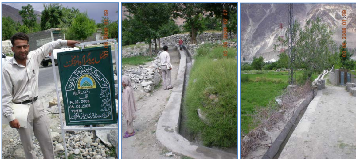
Figure 14: Jutal Bala channel lined under participatory process of Water Management Directorate, Department of Agriculture
