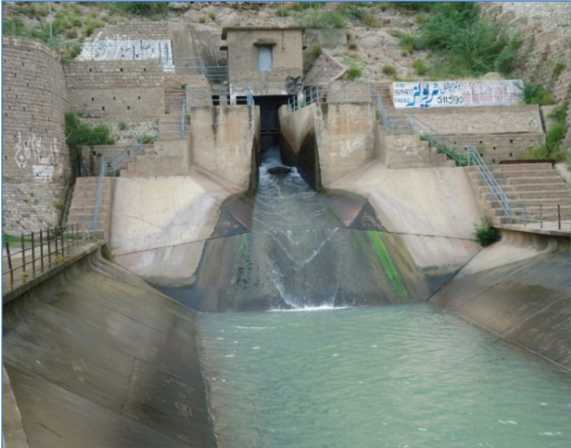
Figure 33: Irrigation canal of the Tanda dam, Kohat District of Khyber Pakhtunkhwa
